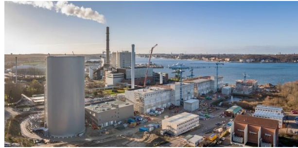
K.I.E.L. coastal power plant: 60-meter-high heat storage unit, engine halls adjacent (© Stadtwerke Kiel AG)
